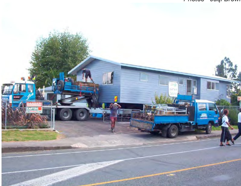
First house getting ready for the move
