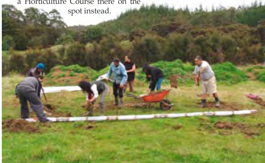
Whanau Students preparing the ground for the erection of a Hot-House
